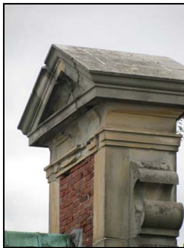
East Transept Gable Pediment
