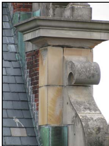
East Transept Gable Pediment and Roof
