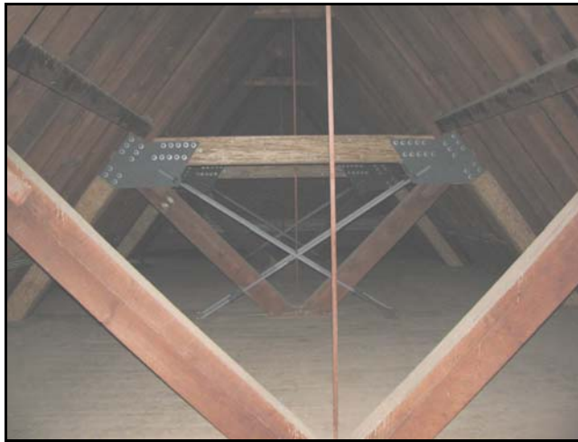
Completed Truss Work in Attic
